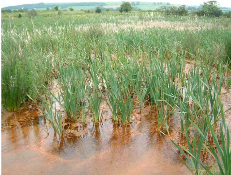
Figure 3.2. Ferruginous mine water entering a recently-commissioned aerobic wetland system at St Helen Auckland 13 , County Durham, UK.
